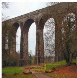
Top label: viaduct
